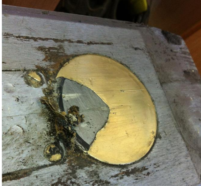
Fig.15. Pressure cell protective shell damage
